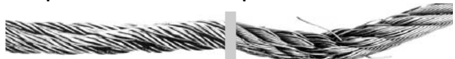
Crushing. Because of loose winding on drum, rope was pulled in between underlying wraps and crushed out of shape.
