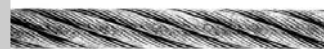
Excessive exposure to elements. Too much exposure combined with surface wear and loss of lubrication caused corrosion and pitting.
