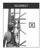
Only the energy absorbing end of the lanyard is to be connected to the dorsal attachment D-ring of a full body harness. The non-energy absorbing end should be connected to the anchorage connector. Never use additional energy absorbers or energy absorbing lanyards, if one is already attached to the subsystem.
